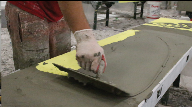
EIFS SYSTEM INSTALLATION
