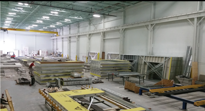
STEEL FRAME ASSEMBLY
